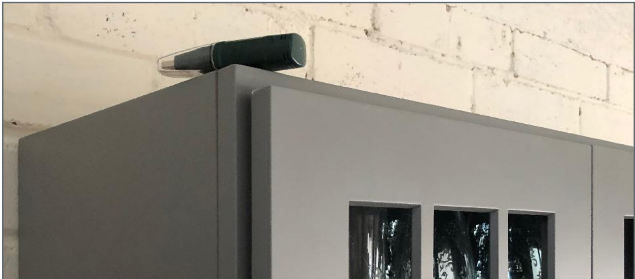
Image17: One of the data loggers installed in the Great Room.
