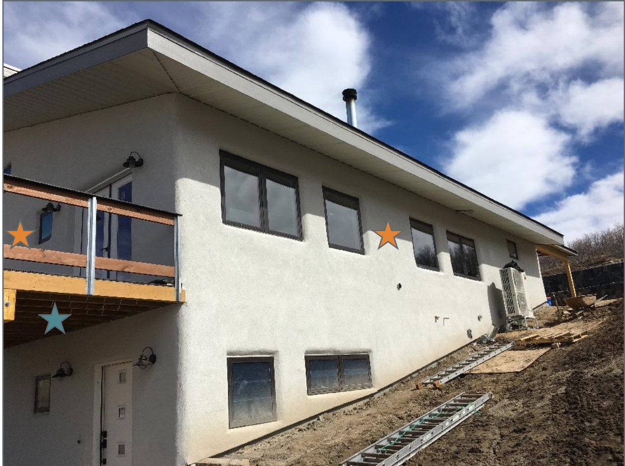
Image 12: View of the South and West walls of the building (respectively: right and left). The stars indicate the approximate locations of the embedded sensors (orange), and the ambient data logger under the deck (blue).
