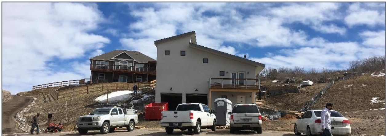
Image 04: View of the West elevation of the building.
